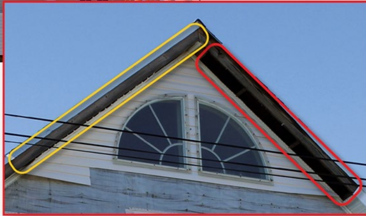
The inset shows the remaining exposed soffit edge on the left side of the ridge (yellow outline) and missing vinyl soffit panels on the right side of the ridge (red outline).
