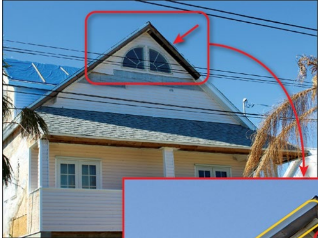
The inset shows the remaining exposed soffit edge on the left side of the ridge (yellow outline) and missing vinyl soffit panels on the right side of the ridge (red outline).
