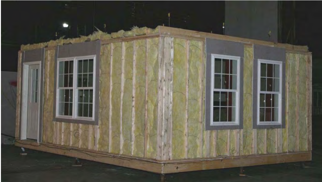
Figure 4: Room exterior walls (south and east walls).
