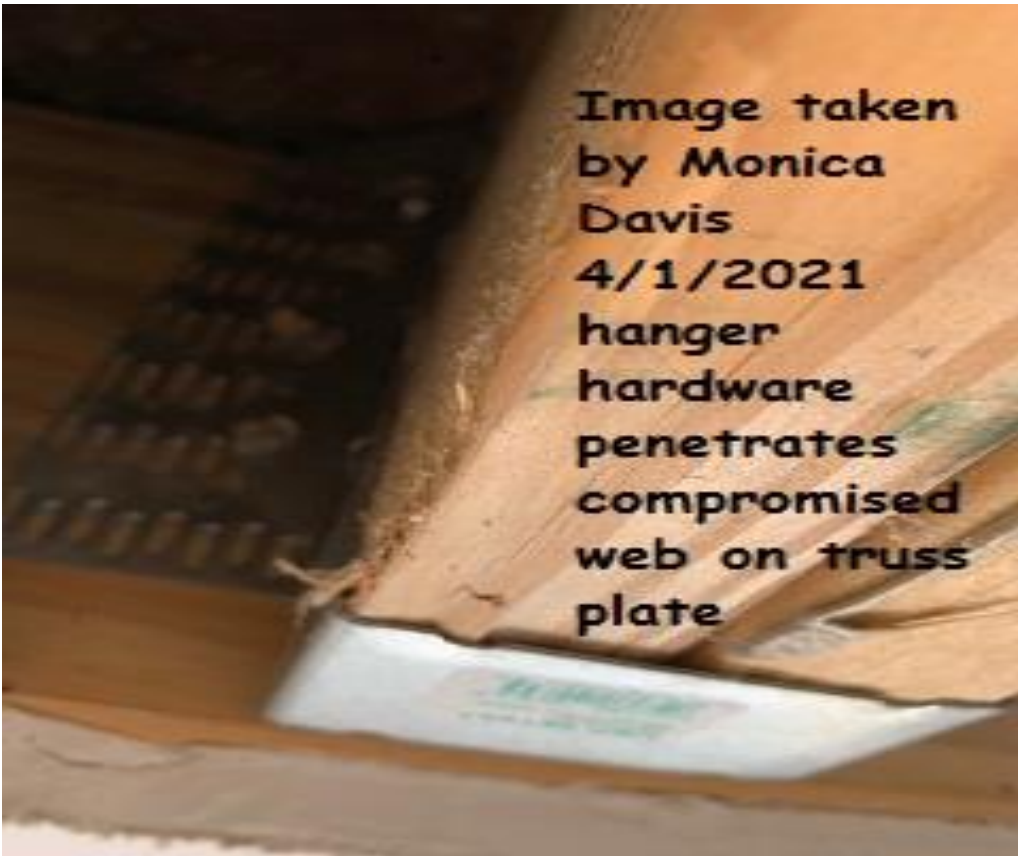
Image taken by Monica Davis 4/1/2021 image shows truss in hanger with 1 1/2 nails here 3 inch screws belong and gap in hanger is a quarter of an inc
