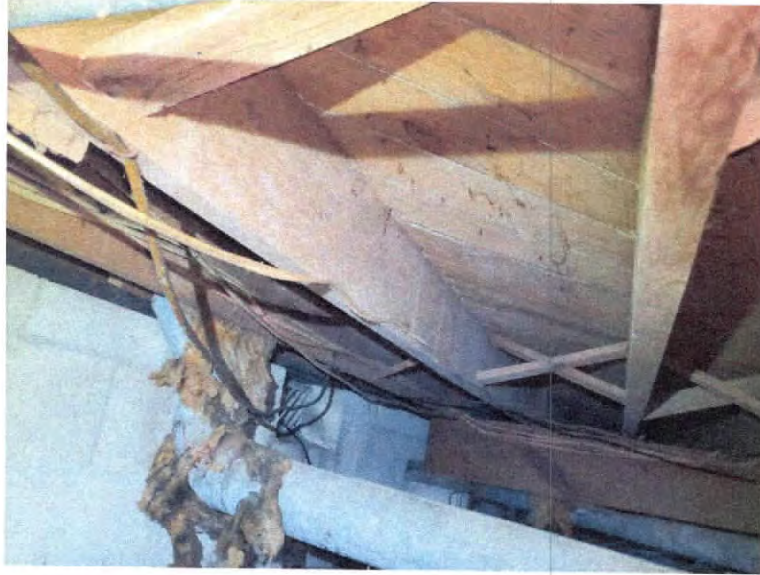
Figure 6 Floor Joists and Foundation wall
