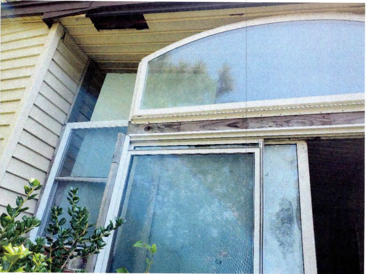
Figure 1 – Front Porch Entrance
