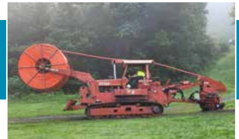
Fiber installation underway in Shenandoah County.
