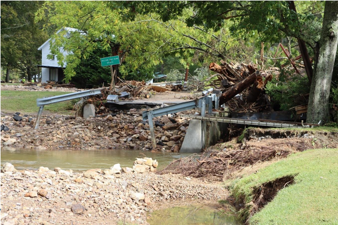
Figure 5: Destroyed Bridge in the City of Bristol
