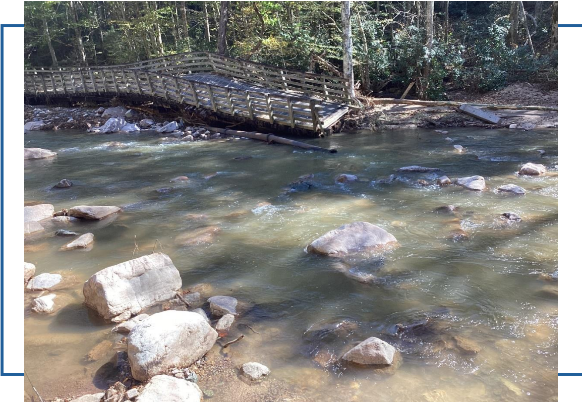
Figure 7: Creeper Trail Destruction in the Town of Damascus
